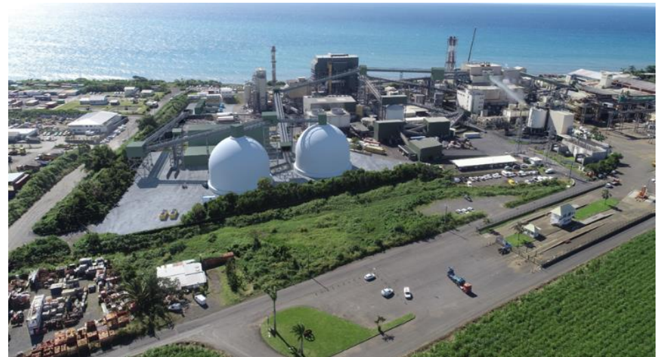
Projected integration of the new biomass storage domes on Bois-Rouge plant site
