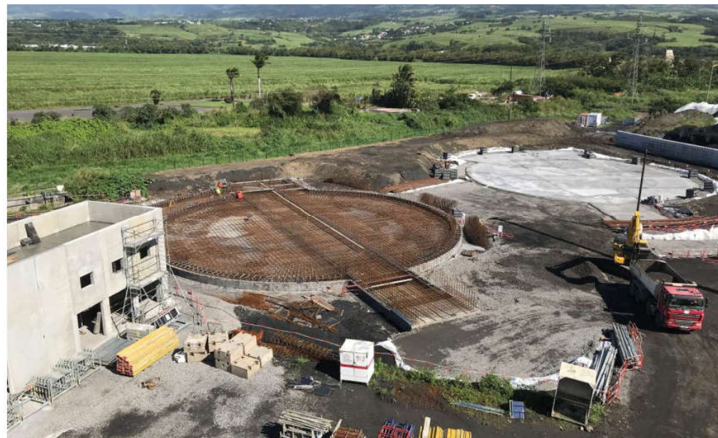
Overview picture of the biomass storage domes foundations
