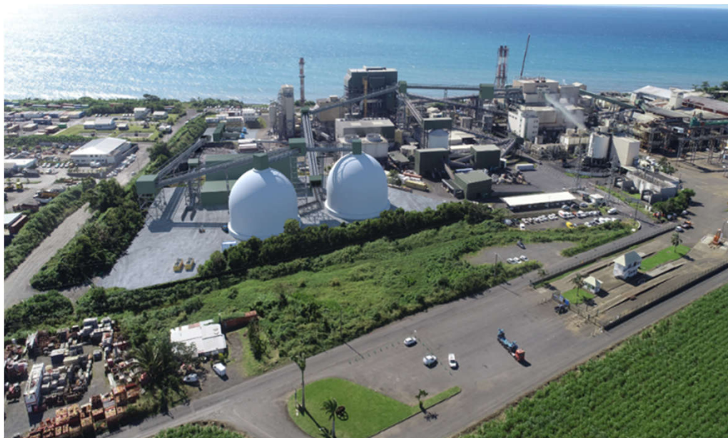
Projected integration of the new biomass storage domes on Bois-Rouge plant site
