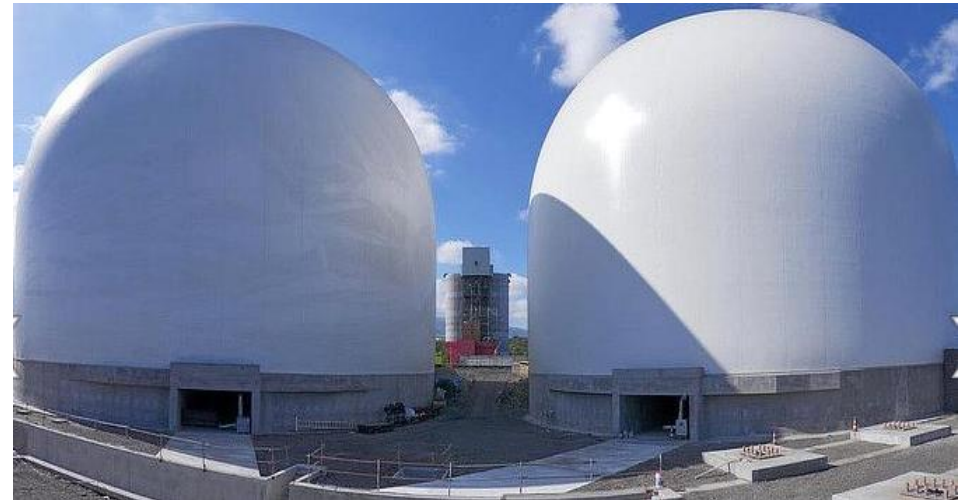
Picture of the biomass storage domes
