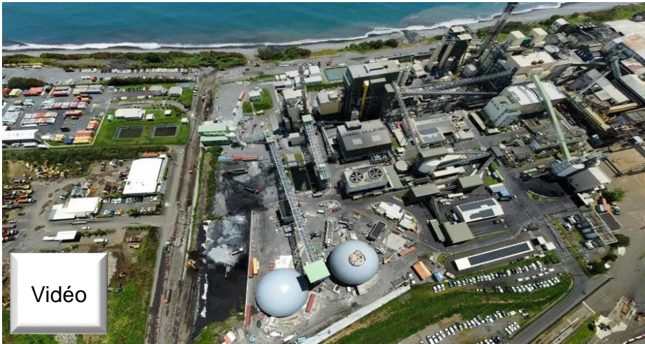
Integration of the new biomass storage domes on Bois-Rouge plant site
