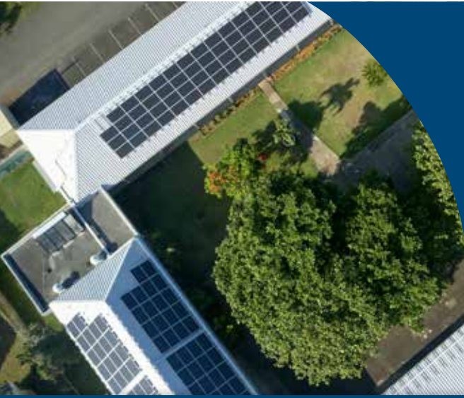
Self-consumption solutions and private electricity sales agreements - PPA -
