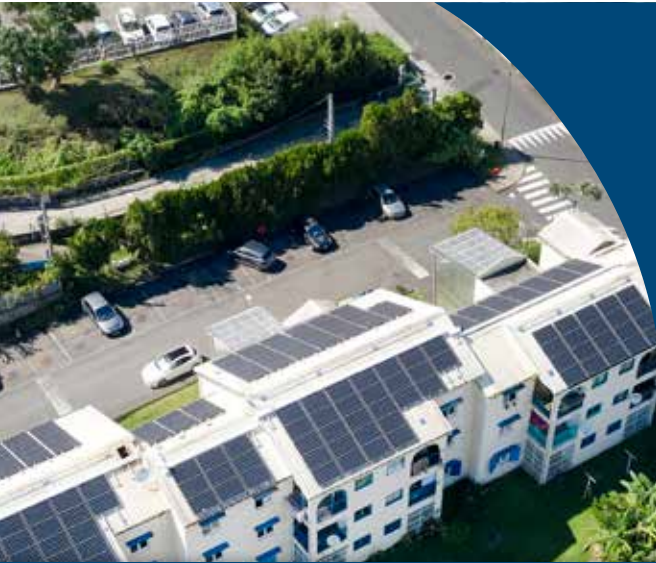
Enhancement of property assets through roof renovation - asbestos removal and compliance -
