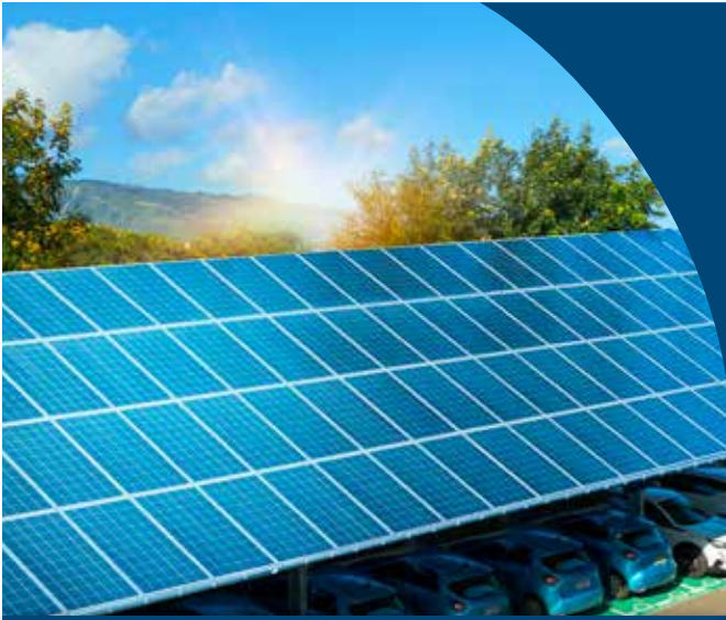
Installation of solar car park canopies
