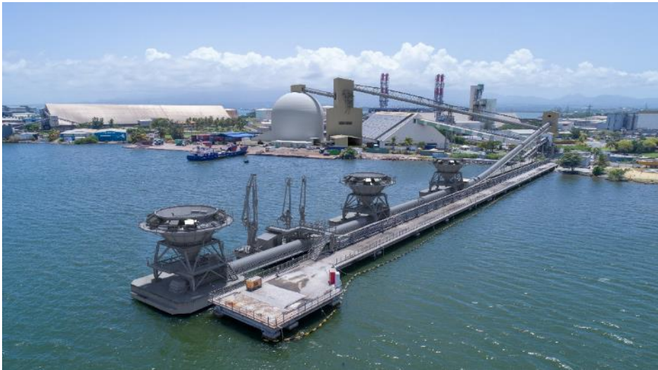
Biomass storage dome on the port of Pointe-à-Pitre (Guadeloupe)
